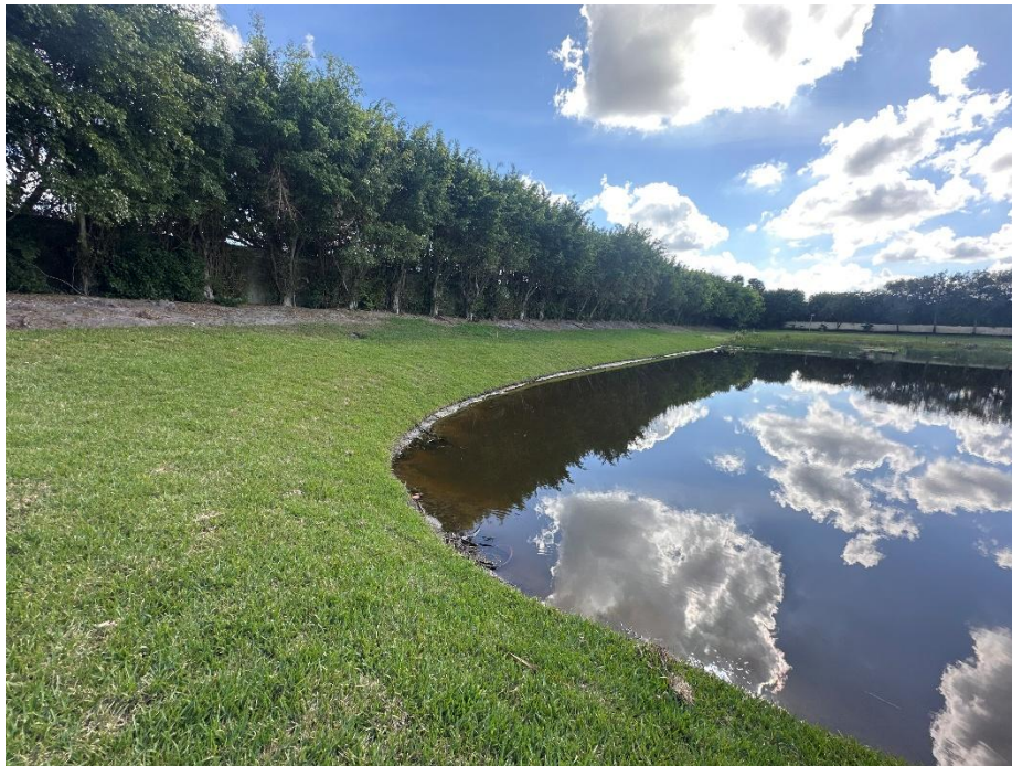
Figure 3. Turf Reinforcement Mat installed in Delray Beach, Florida
